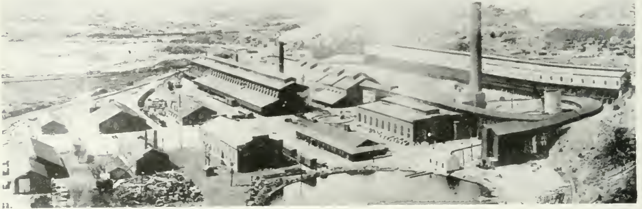
Fig. 68—General View of Copper Cliff Smelting Plant.
